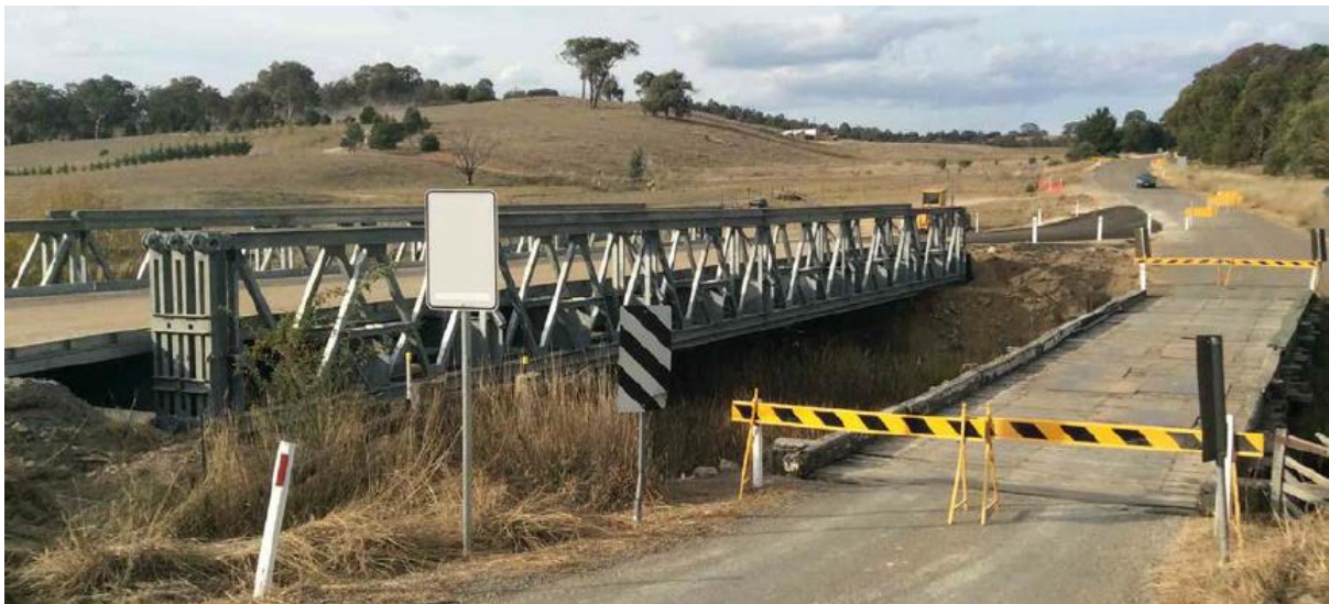
Figure 3. A typical LOC modular steel trussed bridge
